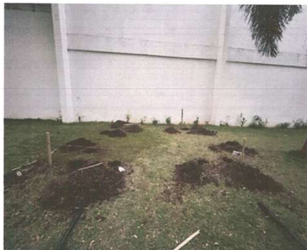
Centerline marking and excavation pits.
