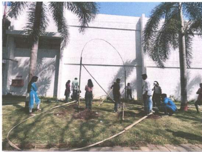
Placing of Arches in the excavation pits.
