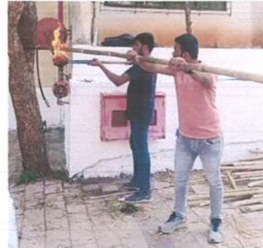
Heating bamboo with Flame torch
