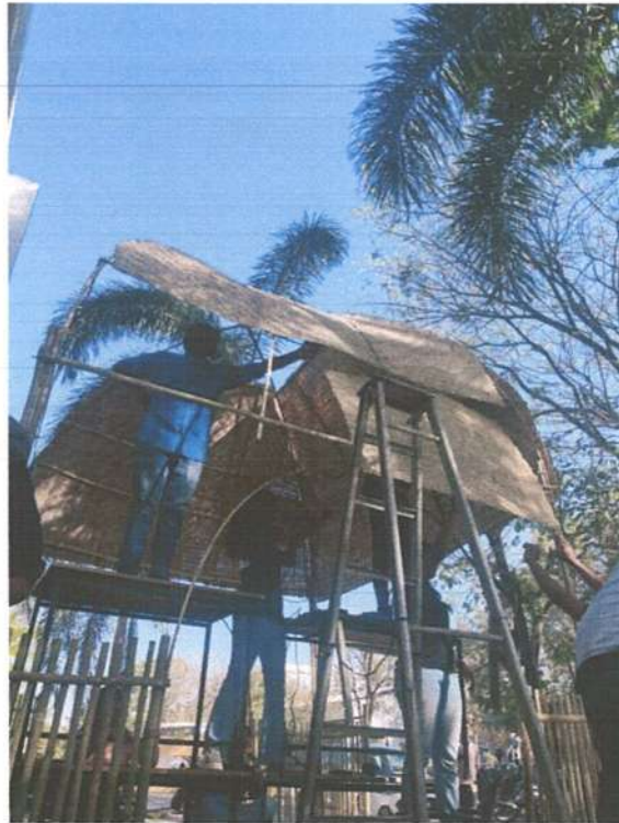
Fitting of bamboo mats for roofing.
