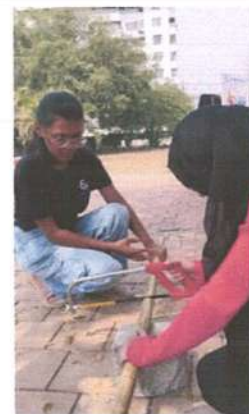
Cutting of Bamboo using a hacksaw
