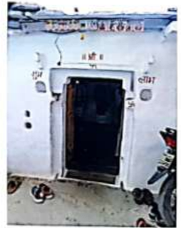
Door - Height of doors is small (1.2-1.5) to get + diffused light
