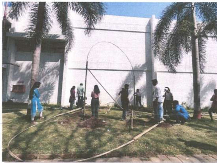
Placing of Arches in the excavation pits.
