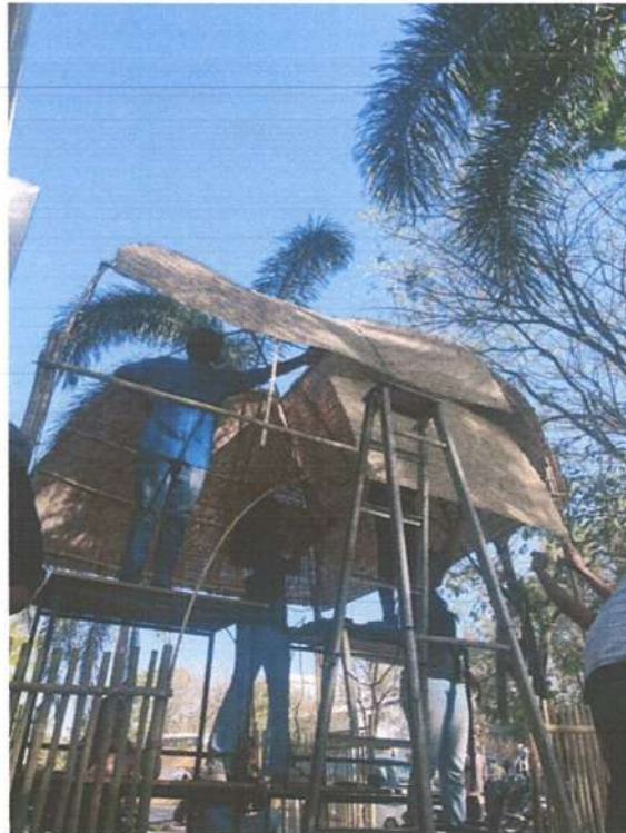
Fitting of bamboo mats for roofing.
