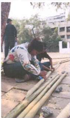
Marking of bamboo using tape
