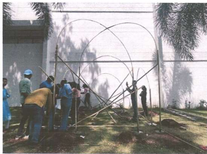
Joining the framework and giving temporary support to the framework for stability.
