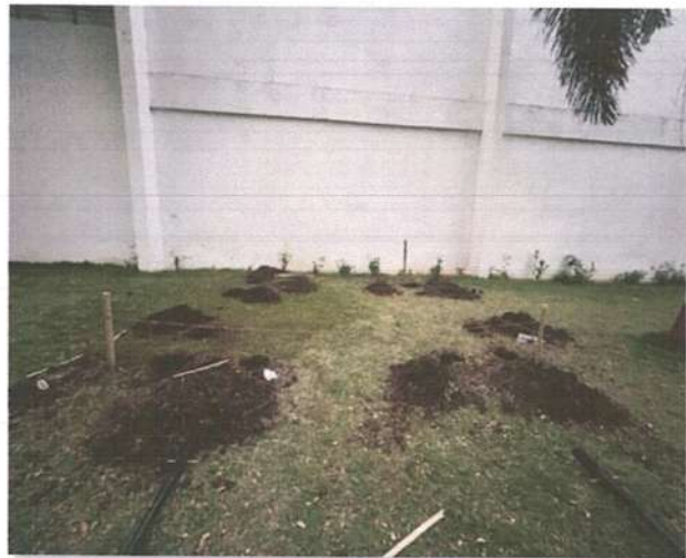
Centerline marking and excavation pits.
