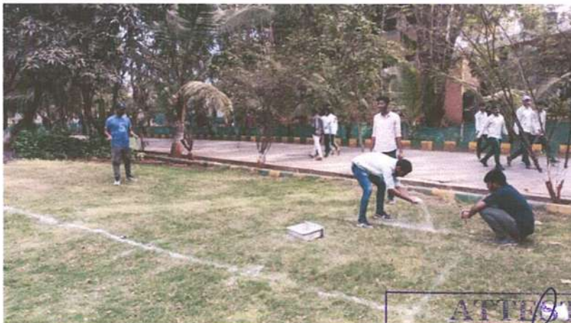
Centre Line Marking
