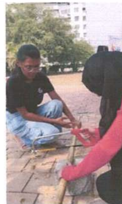
Cutting of Bamboo using a hacksaw
