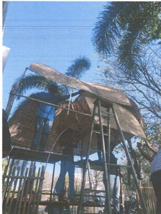
Fitting of bamboo mats for roofing.
