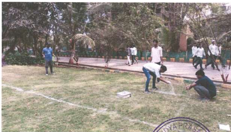
Centre Line Marking
