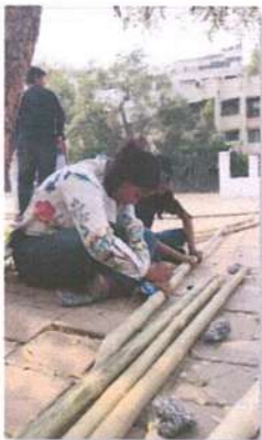
Marking of bamboo using tape
