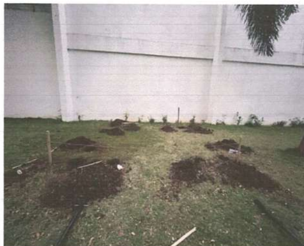
Centerline marking and excavation pits.
