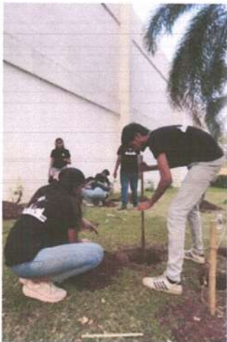
Digging site with the help of L-shaped steel rods.
