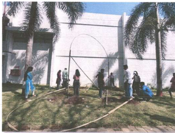
Placing of Arches in the excavation pits.
