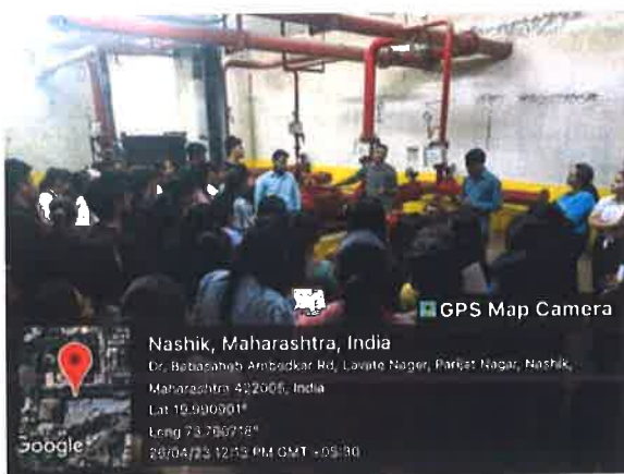
Visit to City Centre Mall for Fire Fighting Services
