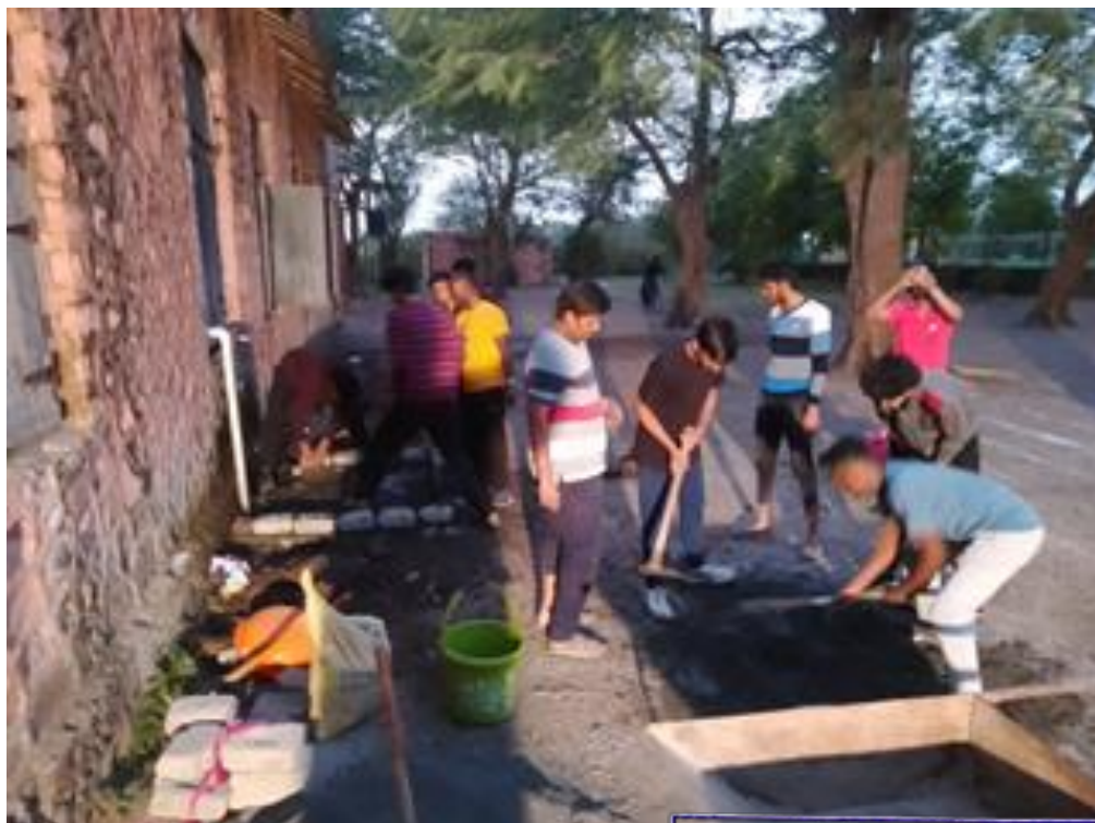
Soak Pit construction by NSS candidates.
