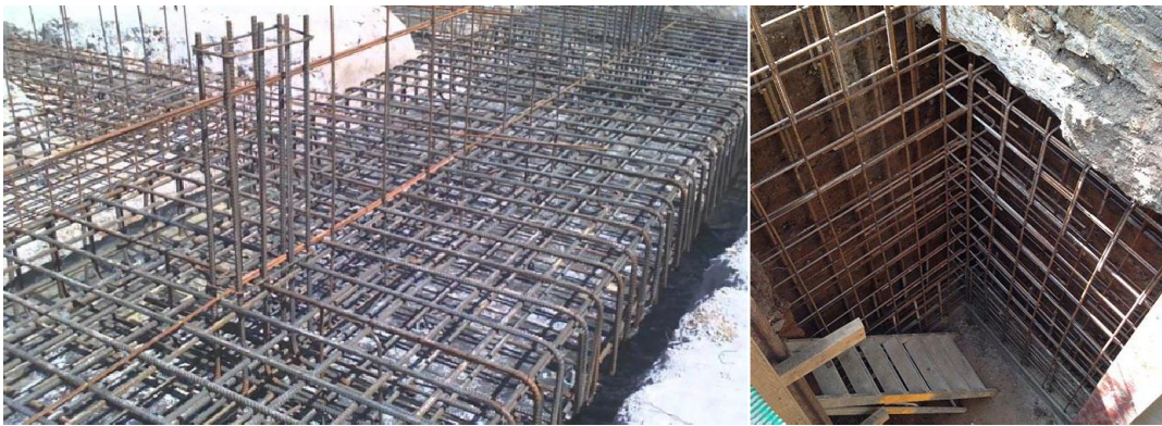
Box excavation done and reinforcement ready for raft slab ready at a construction site
