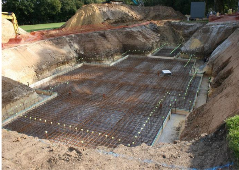
Box excavation done and reinforcement ready for raft slab ready at a construction site
