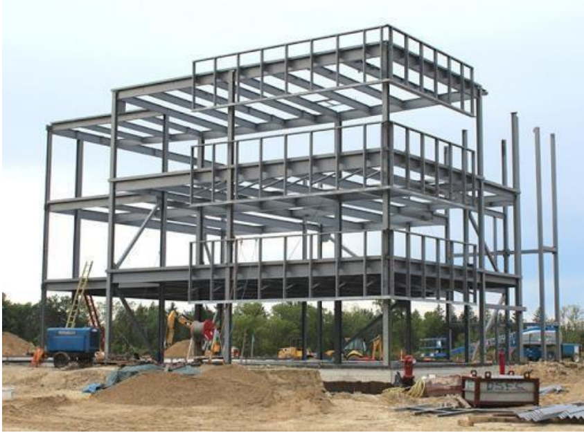
Steel construction and metal decking for multi-level building
