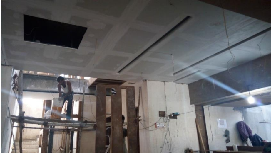
Constriction Details on site
