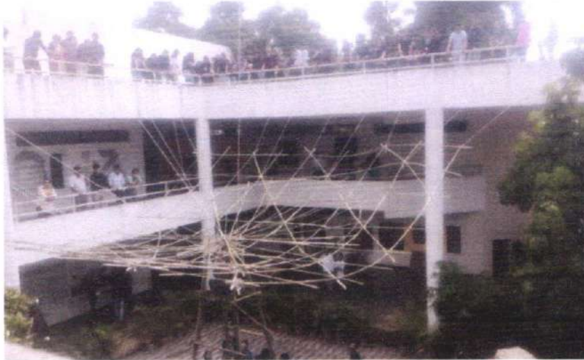
Students installing mushroom column for courtyard
