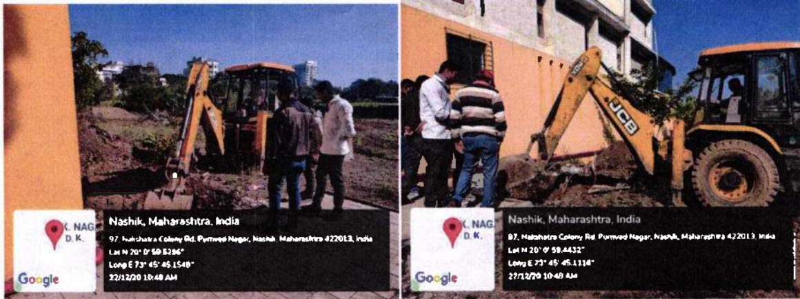
Rain Water harvesting Pit 1 (Terrace rain water) Excavation
