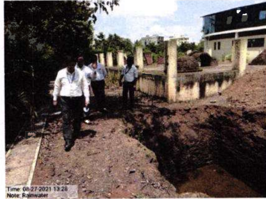
Rain water harvesting pit 2(Surface rain water collection) Excavation
