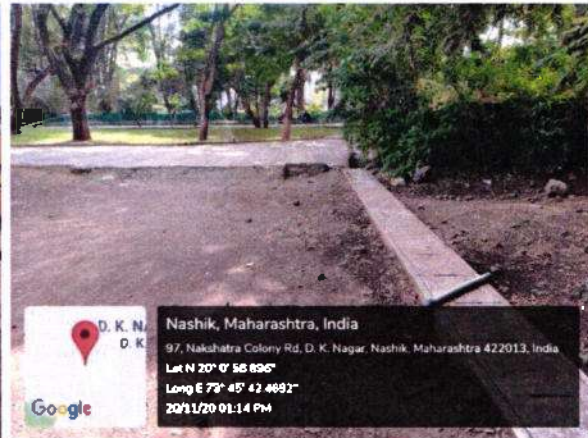
Channels for rain water collection from surface water in the campus to recharge pit
