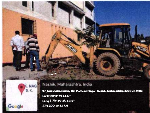
Rain Water Pit 1 (Terrace rain water) Excavation
