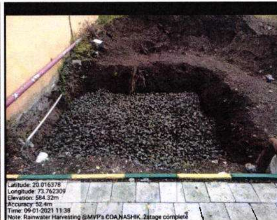
Rain water harvesting pit 1 (Terrace rain water) refilling with granular material
