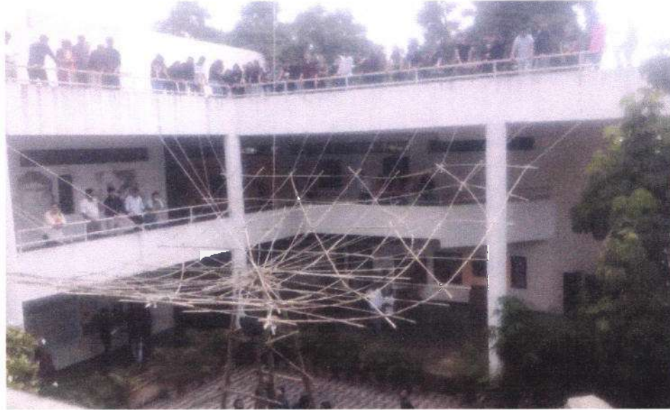
Students installing mushroom column for courtyard
