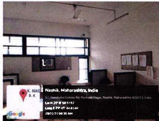
CCTV in Staff room
