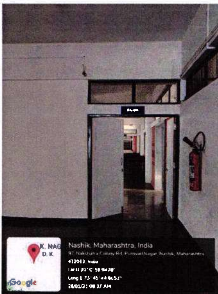
CCTV in Common passage area
