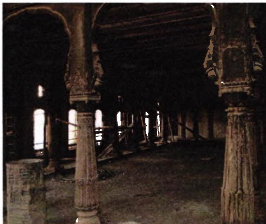
Old wooden columns at Sarkarwada, Nashik
