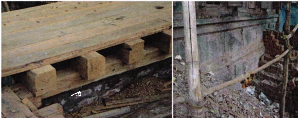
Restoration work at Sarkarwada
