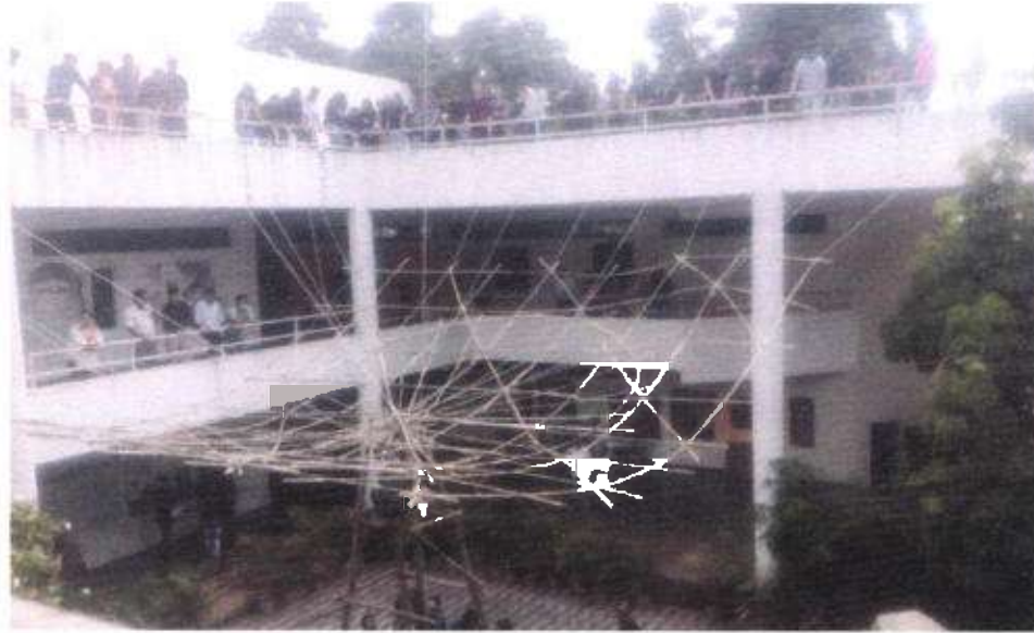
Students installing mushroom column for courtyard
