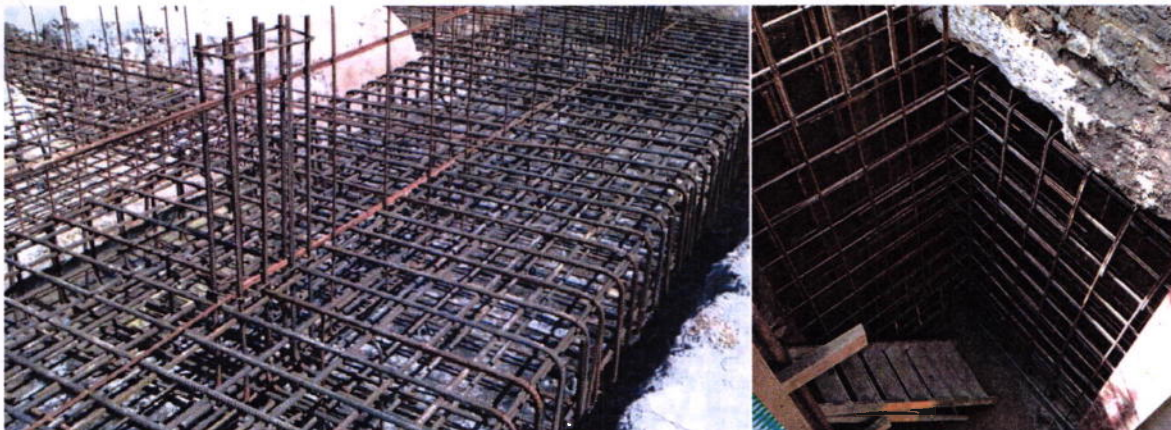
Reinforcement details of raft slab, column junction and Pardi observed on site
