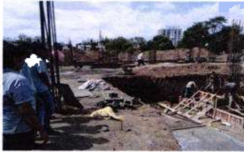
Foundation Formwork
