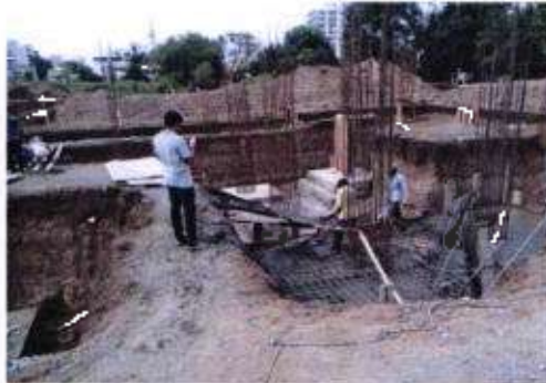
Concreting at Footing
