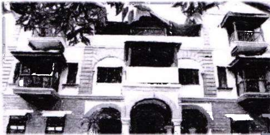
Front Elevation of structure
