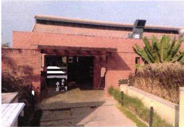
Exterior View of resort
