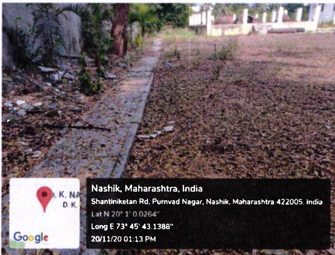
Channels for rain water collection from surface water in the campus to recharge pit
