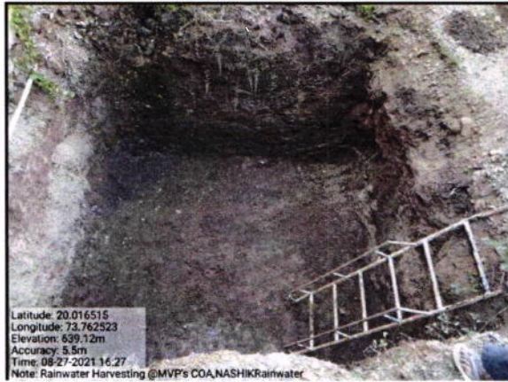
Rain water harvesting pit 1 (Terrace rain water) refilling with granular material
