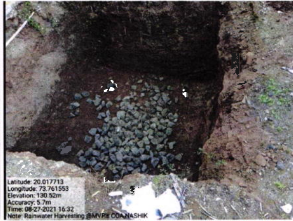
Rain water harvesting pit 1 (Terrace rain water) refilling with granular material
