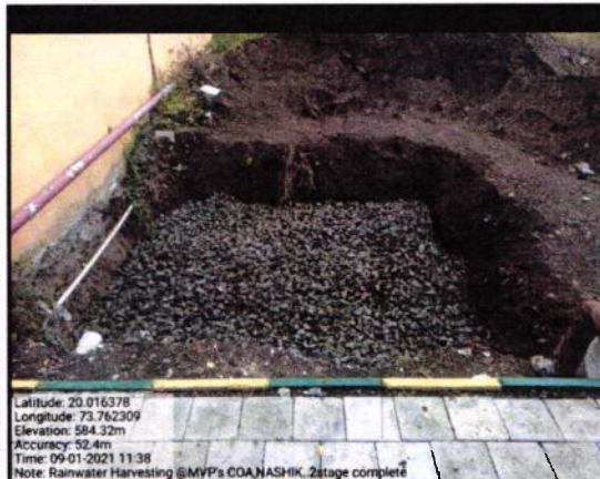
Rain water harvesting pit 1 (Terrace rain water) refilling with granular material
