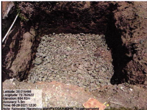
Rain water harvesting pit 1 (Terrace rain water) refilling with granular material
