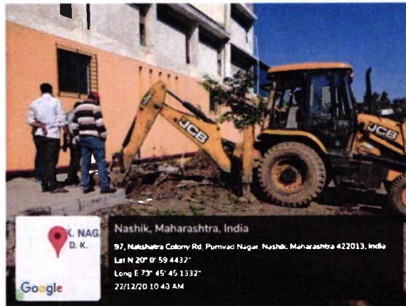
Rain Water Pit 1 (Terrace rain water) Excavation
