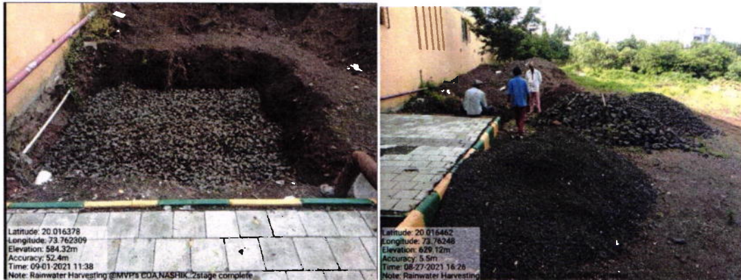
Rain water harvesting pit 1 (Terrace rain water) refilling with granular material
